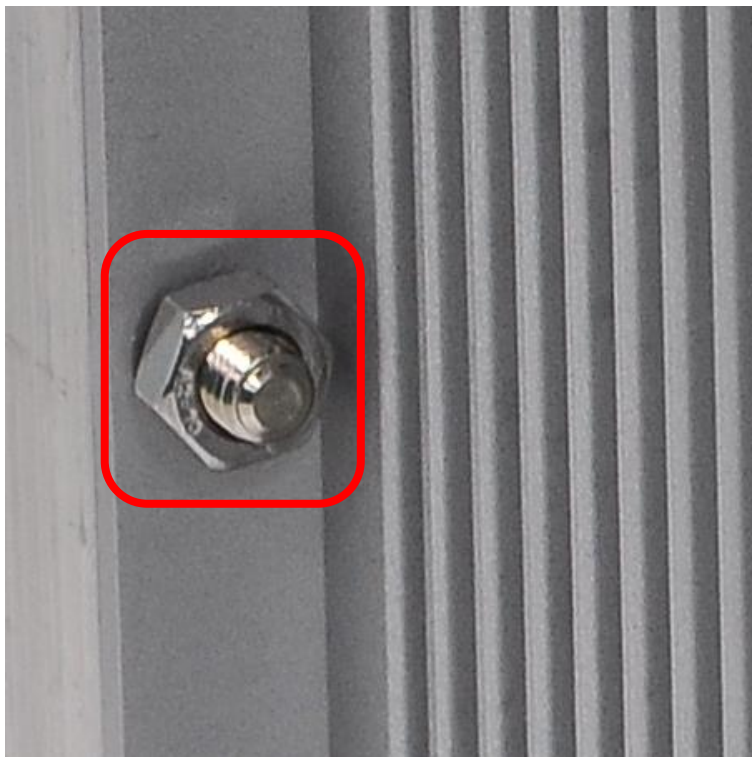
Ground screw of the switch
