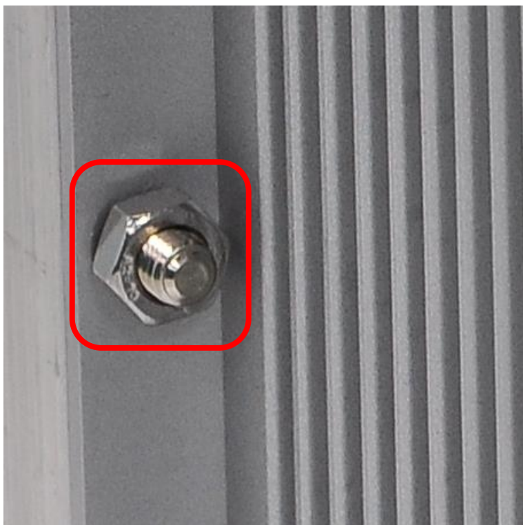
Ground screw of the switch
