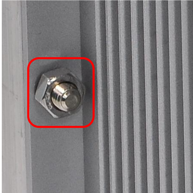
Ground screw of the switch
